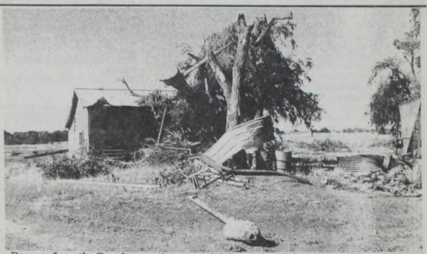
Damage from the Tuesday evening storm left Larry Don Price's barn a heap of twisted metal.
