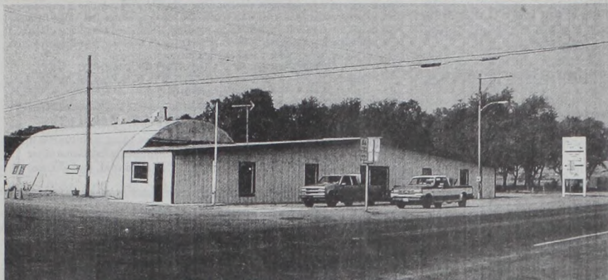
The Valley Farm Store in Quitaque has been working hard on their expansion and remodeling efforts to better serve their customers in the Valley Region. Stop by and check it out!
