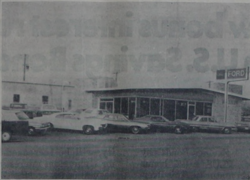
MULLINS FORD CO.—This modern automobile sales and service center serves a wide territory around Turkey—From Memphis west to Tulsa. It's well stocked display of new and used cars and pickups, comfortable offices and showroom, parts department and repair and service shop, is a business that Turkey can well be proud of.
