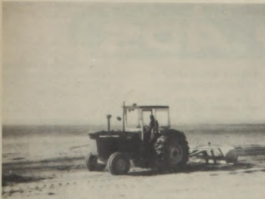
Duke Woods on the Rusty Henson farm, patching a broken terrace.
