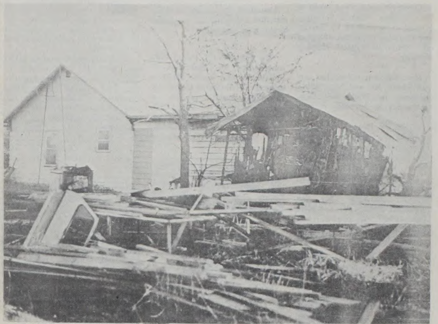
Storage building destroyed by blaze Monday at Allen Greene residence in Turkey.
