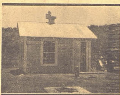
One of the pumping units of the vast Humble Pipe Line system that help to boost oil from the widespread Texas hinterland to the coast.
