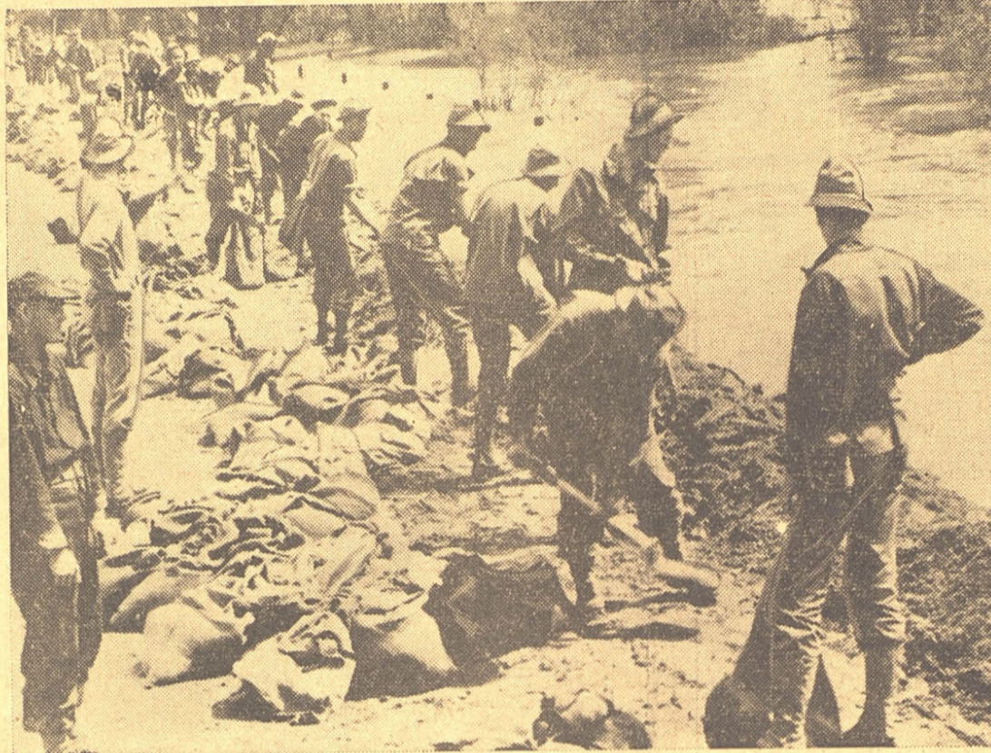
ENGINEERS BATTLE FLOOD—U. S. Army Engineers build levee to stem rising crest of Boise River overflowing bottom lands near Gowen Field, Idaho. More than 150 families were evacuated from their homes. Flood threatened many bridges.
