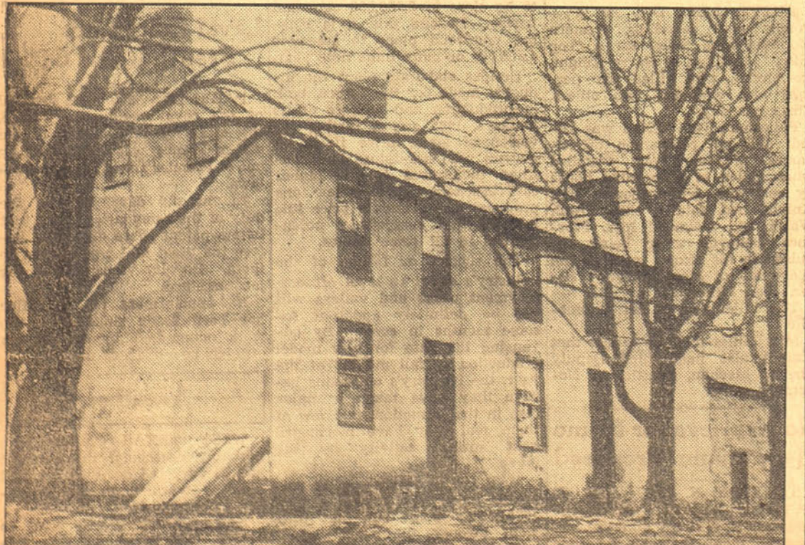
This dilapidated house, hidden in the woodlands of Bucks county, Pa., yielded evidence to indicate it was the hideout of the kidnapers of Caleb Milne IV, scion of a wealthy Philadelphia family. The house is about three miles from the spot on the highway, near Doylestown, Pa., where young Milne, bound, gagged and drugged, was found suffering from exposure. (Associated Press Photo)
