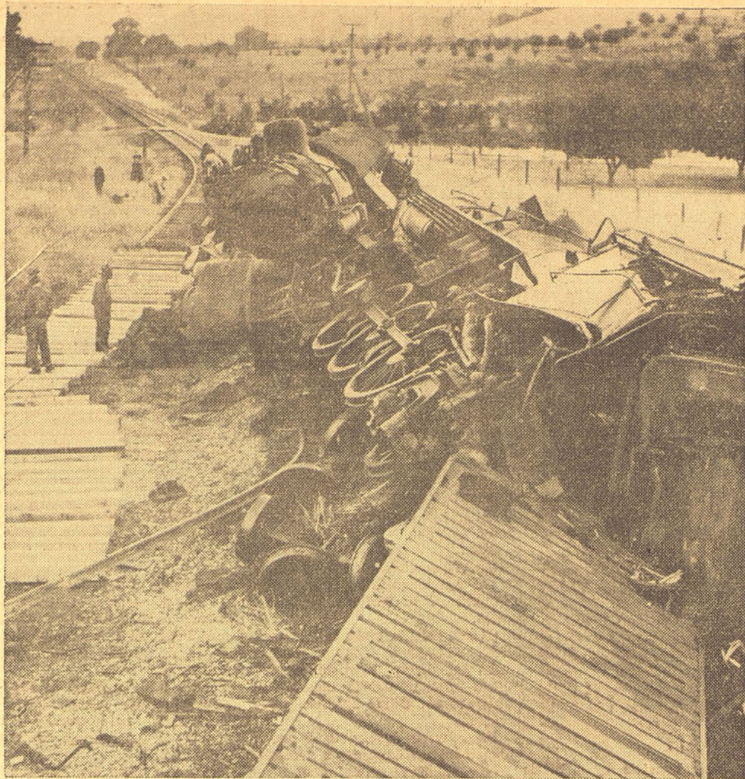
HEAD-ON CRASH RESULT —Here is what happened when a heavy Western Pacific freight locomotive, without cars, collided head on with the Exposition Flyer, passenger express, near Livermore, Cal. Three were killed and eleven injured. Workmen lay emergency track.
