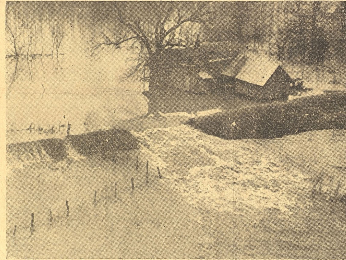
Thousands of residents have been forced to move to high ground as a result of breaks in the Stephen-Kael levee on the White river near Newport, Ark. NEA's photographer
