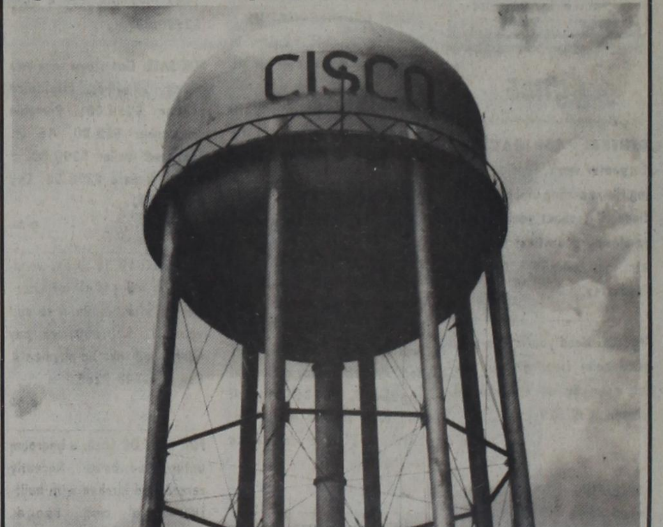
A BEFORE SHOT of Cisco's water tower shows how the tower used to look before it was sandblasted on the outside and inside and repainted. In this photo some of the old silver paint had already been sandblasted from around the bottom part of the tower reservoir. (staff photo)
