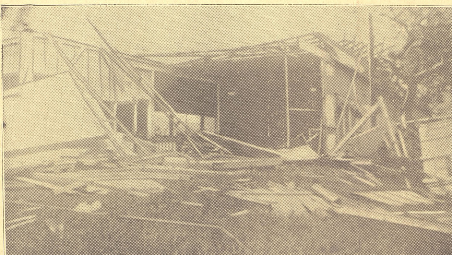
These two pictures were taken in the stricken Texas valley district just after the disastrous storm which killed at least 100 persons and injured hundreds more, swept entire towns and completely cut off communications. These pictures, taken near Port Isabel, northeast of Brownsville, were rushed by auto over almost impassable roads to Corpus Christi and then sent to Dallas by plane. In the above photo men may be seen hunting for bodies. The lower picture shows a wrecked building.
