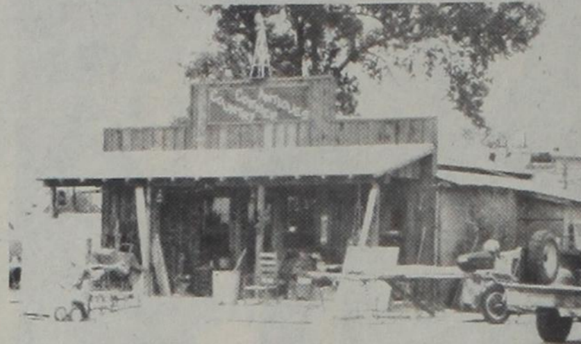
NEW LOOK—Country Corner Antiques, at the "Y" on Hwy. 80 West has a new look after their remodeling. A new exterior to the front of their building gives the business an old time general store charm. (Staff Photo)
