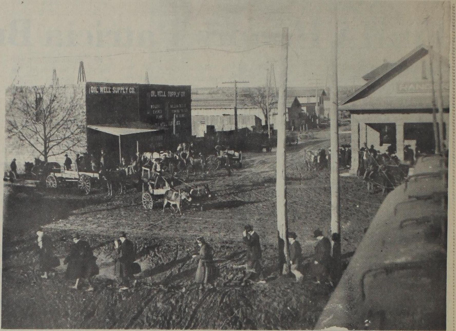
The Building On The Left Is Now The Ranger Lumber Yard.
