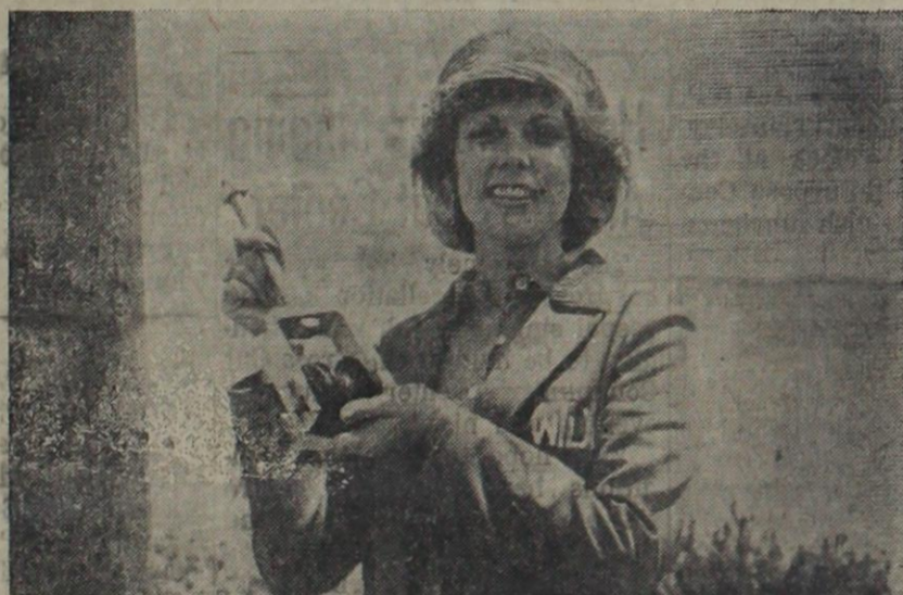
This insulator and rack is used to bring your electric service from the utility pole to your home.
