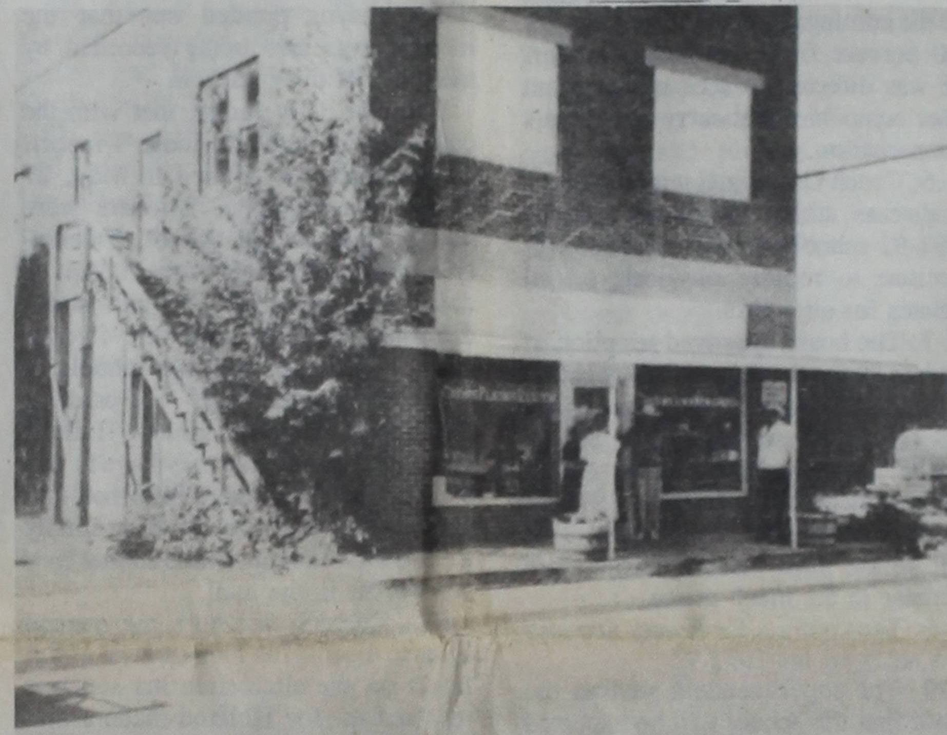
ESTABLISHED IN 1908 — The Cross Plains Review was literally built around some of the printing equipment that still remains intact. A former
