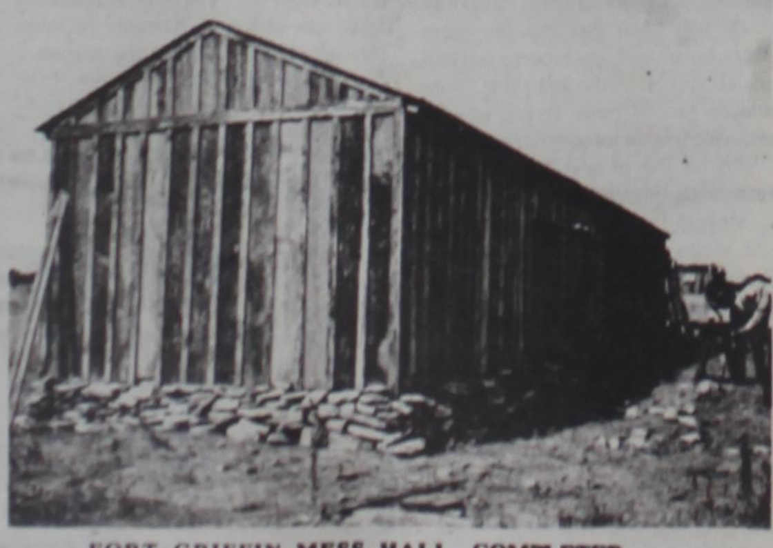
FORT GRIFFIN MESS HALL COMPLETED
