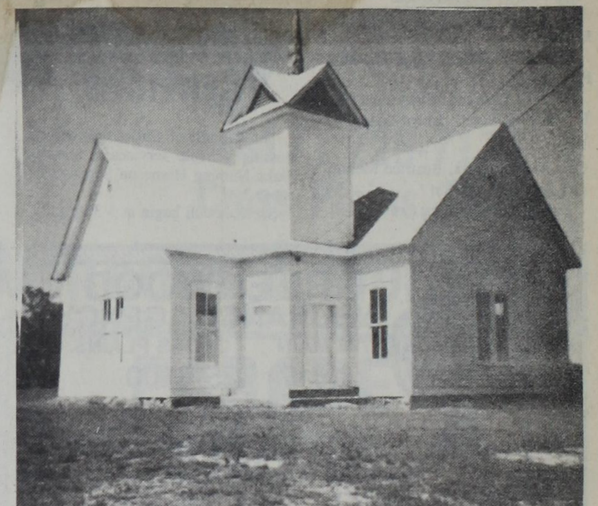
AFTER RESTORATION — The Old Methodist Church at Cottonwood has recently been repaired and painted on the exterior.
