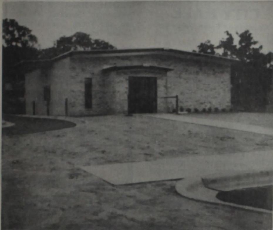
ASSET TO COMMUNITY — The completion of the new City Hall on Main Street is yet another progressive sign in Cross Plains.
