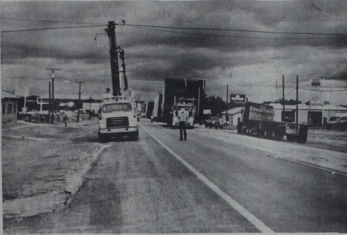
ELEVATING POWER LINES-- A bucket truck is pictured raising power lines for the caravan to pass. (Photos courtesy of Trish Hutton.)
