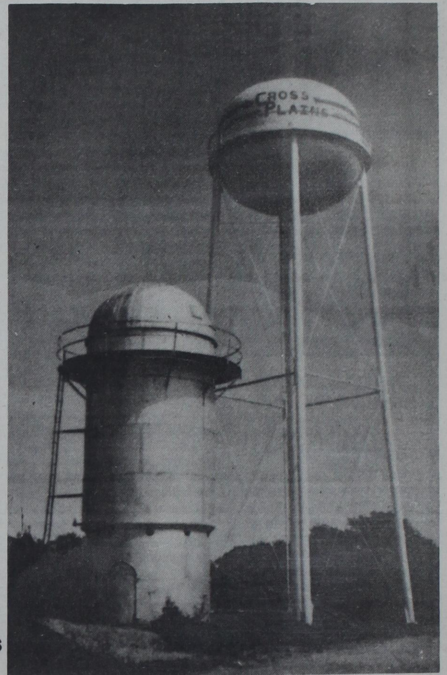
FINISHED PRODUCT — The water tower is now completed with white paint accented with purple and gold trim and lettering.
