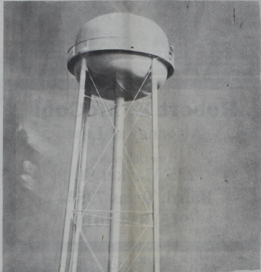
STRUCTURE COMPLETE—Tower stands tall with new coat of white paint.
