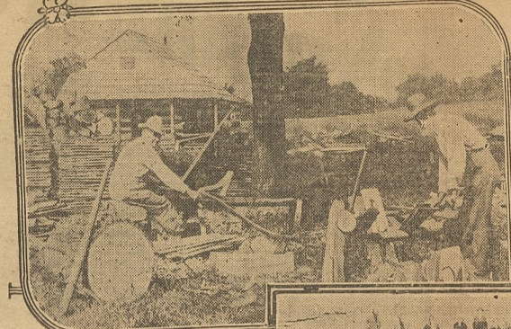
Splitting and shaving shingles—pioneer style—for school house, Sept.-Oct. 1927. Schoenbrunn Memorial Park near New Philadelphia, Ohio. © 1931
