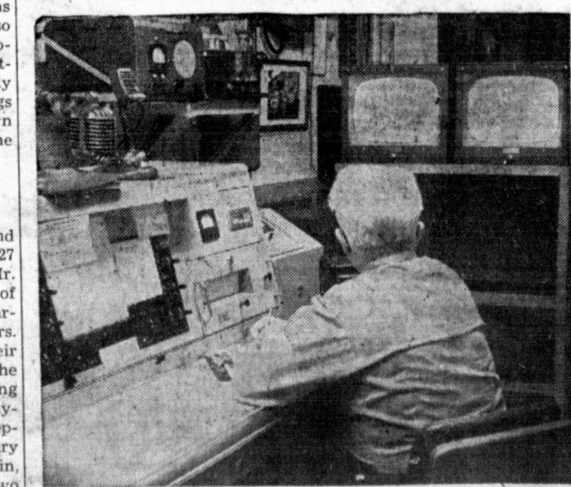
FIRE-WATCHING DELUXE—The Army Ordnance Corps has put television to work spotting fires atop the 29-acre roof of its Clarendon plant. Warm and dry in the protection office, this civilian employee can control the cameras and sound an alarm with the flip of a switch. He replaces four guards at a saving of $21,000 annually.
