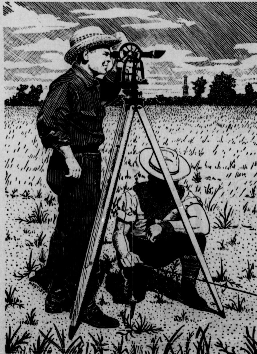
United Gas survey crew lays out a right-of-way for a new United Gas pipe line
