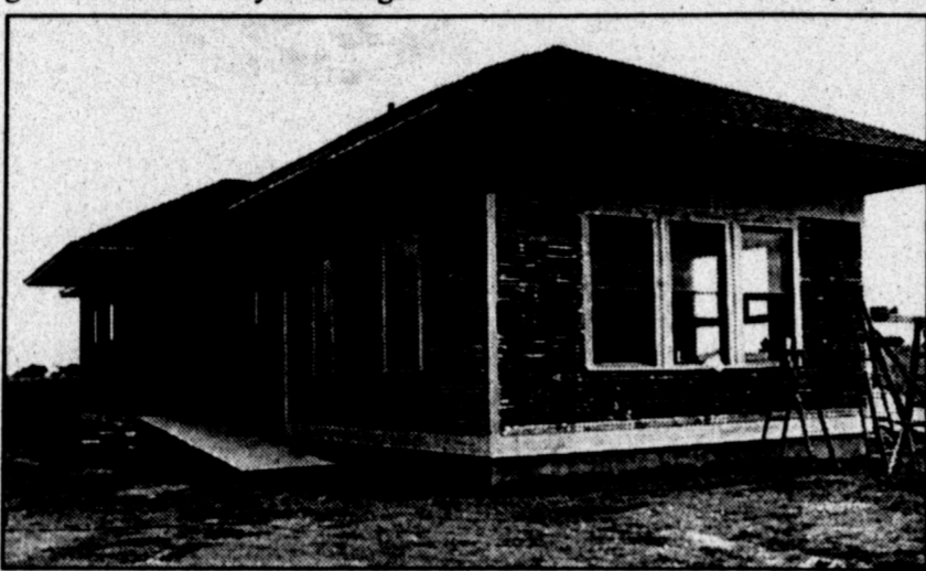
The old depot building is looking better and better thanks to the efforts of a few volunteers. James Owens is heading the renovations for the Saints' Roost Museum and hopes to have the building painted for the up-coming Col. Charles Goodnight Chuckwagon Cookoff on Sept. 27. Enterprise Photo.
