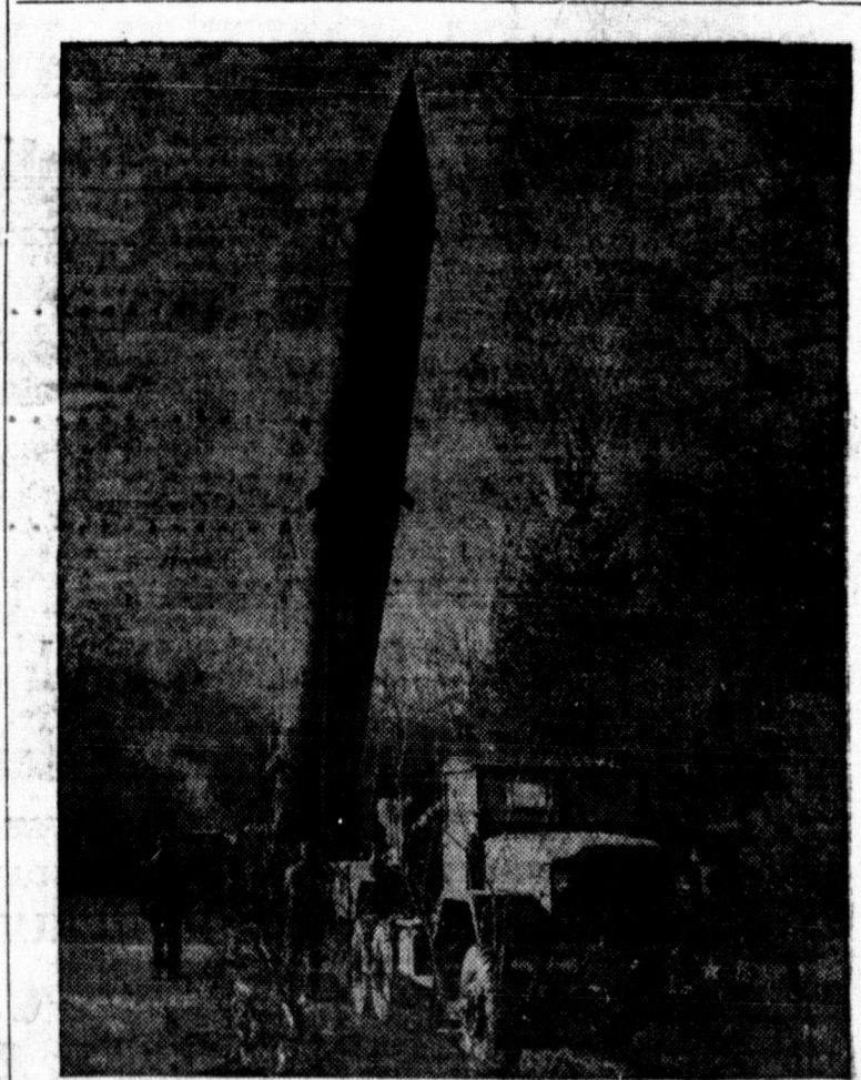
RAISE UP—Using an ordinary winch on the rear of a standard truck, soldiers of the Army's 40th Missile Group raise their Redstone into firing position during a field exercise in Germany. Activated only three years ago, the unit has been in Europe with its 200-mile-range missiles since last summer.
