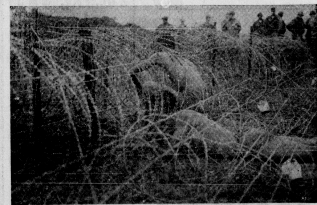
UNDER THE WIRE—Vietnamese soldiers attempt to infiltrate through concertina wire during testing of new techniques for stringing wire obstacles. The obstruction was designed and erected by the 26th Engineer Battalion of the Americal Division near Chu Lai, Republic of Vietnam. Tin cans attached to the obstacle sound an easily identified warning when jiggled. (U.S. Army Photo by Sp4 J. B. Majerus)
