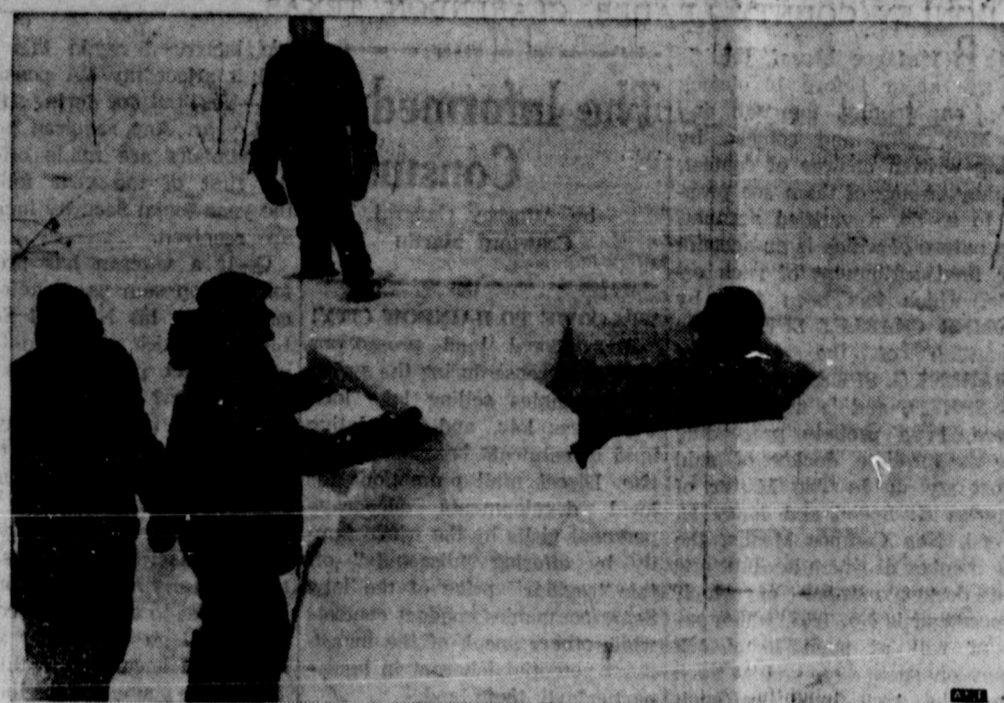
ARMY IGLOO SLEEPS FOUR—Lt. Col. John Todd sets in place one of the last blocks of snow while helping build an igloo at Ft. Richardson, Alaska. Col. Lowell Landre stands inside the structure to guide the final critical blocks into place. The igloo can sleep four or five men and can be used as an emergency shelter in areas where snow building blocks are available. Colonel Landre is head of the U.S. Army Alaska Combat Developments Section (CDS). S/Sgt. Eugene Schreyer and Pfc Ronald Wallace, both from CDS, also took part in building the igloo.
