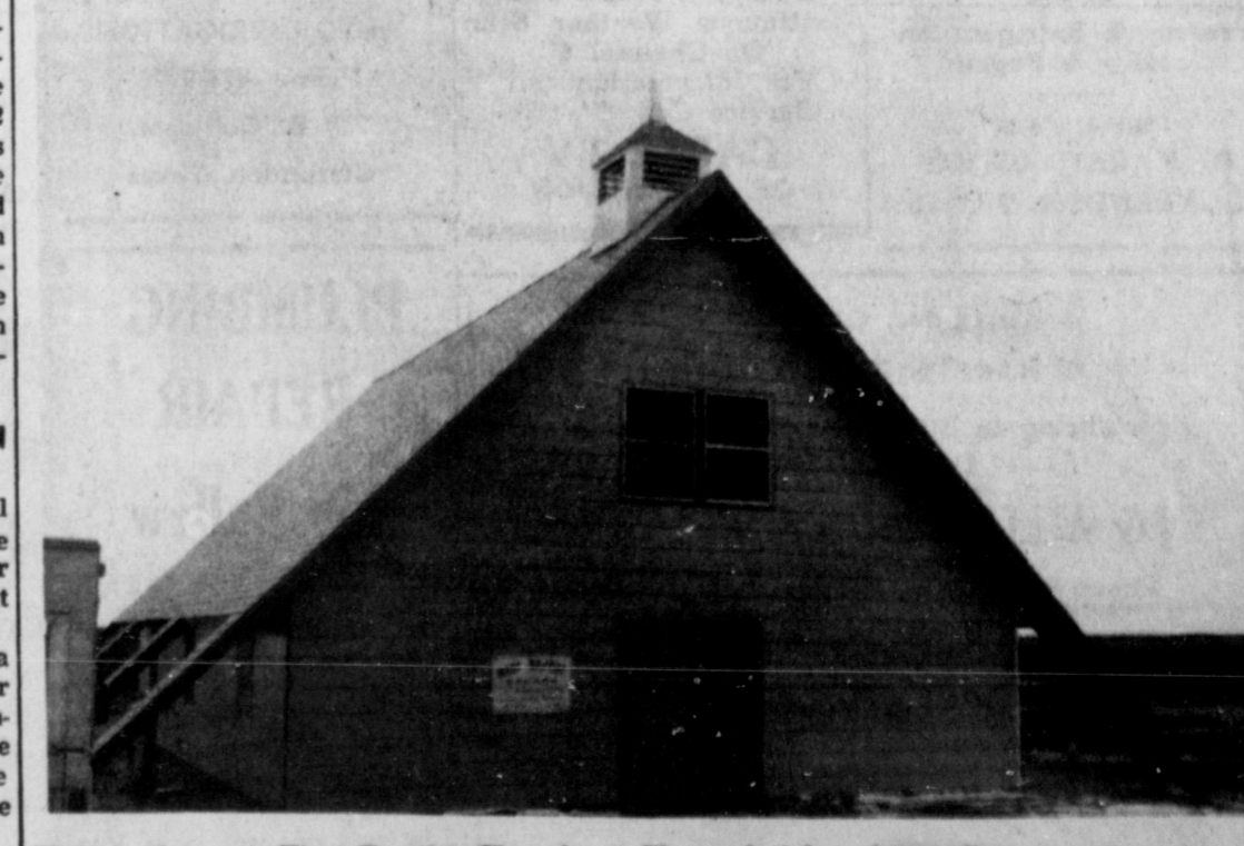
This is the new First Baptist Church at Howardwick where first services were held last Sunday. Construction has principally been done by church members. —Staff Photo
