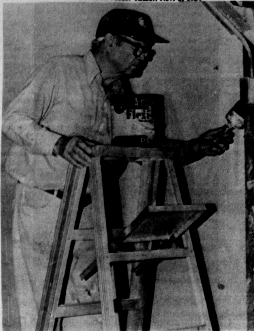
Woody Argo helps paint the walls at the Community Center.
