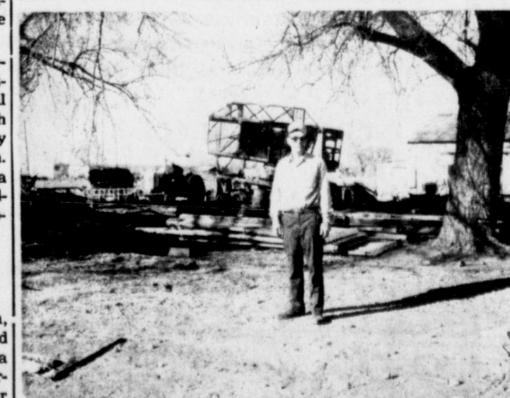
Progress at Lelia Lake — Cecil McAfee, owner of Cecil's Welding and Machine, is standing on the location where his new 40 x 60 welding shop building will be constructed. Behind him is all the steel etc. needed to finish the building. Carl Morris with Morris Sand and Gravel, will pour the foundation and floor. Staff Photo
