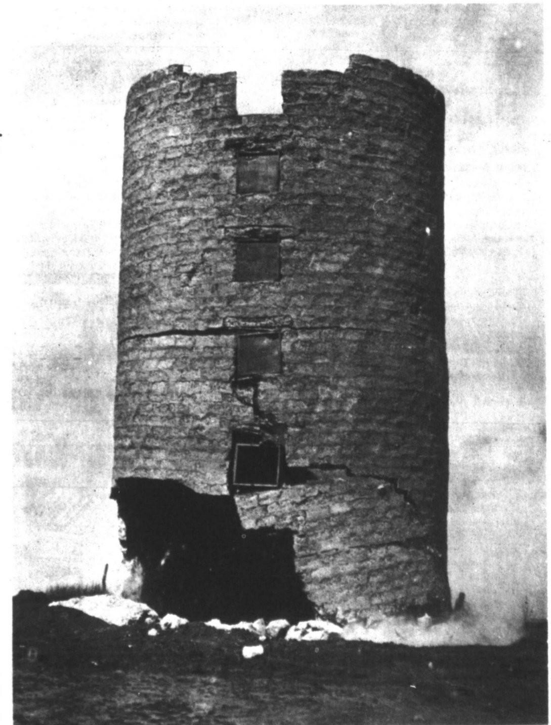
Martin Community landmark bites the dust to make way for irrigation works that may keep the dust settled a good deal better there. Built in 1915 or 1916 by the Speed Brothers of solid concrete block construction on the old Goodnight property on the line between production land owned by Bob Cole and Warren Hardin, the "Old Silo" at Martin was long a landmark near Crossroads. Its twin abandoned structure was torn down by workmen with chisels stone by stone in the depression years, but the property owners either decided that was too expensive or the laborers decided they weren't that hungry. This silo remained till parts of the wall were pulled out by a dozer, breaking several oil rig cables in the process. Removal of the structure will enable the quarter-mile irrigation wheel rig used on the land to travel further before having to be disassembled and turned around.
