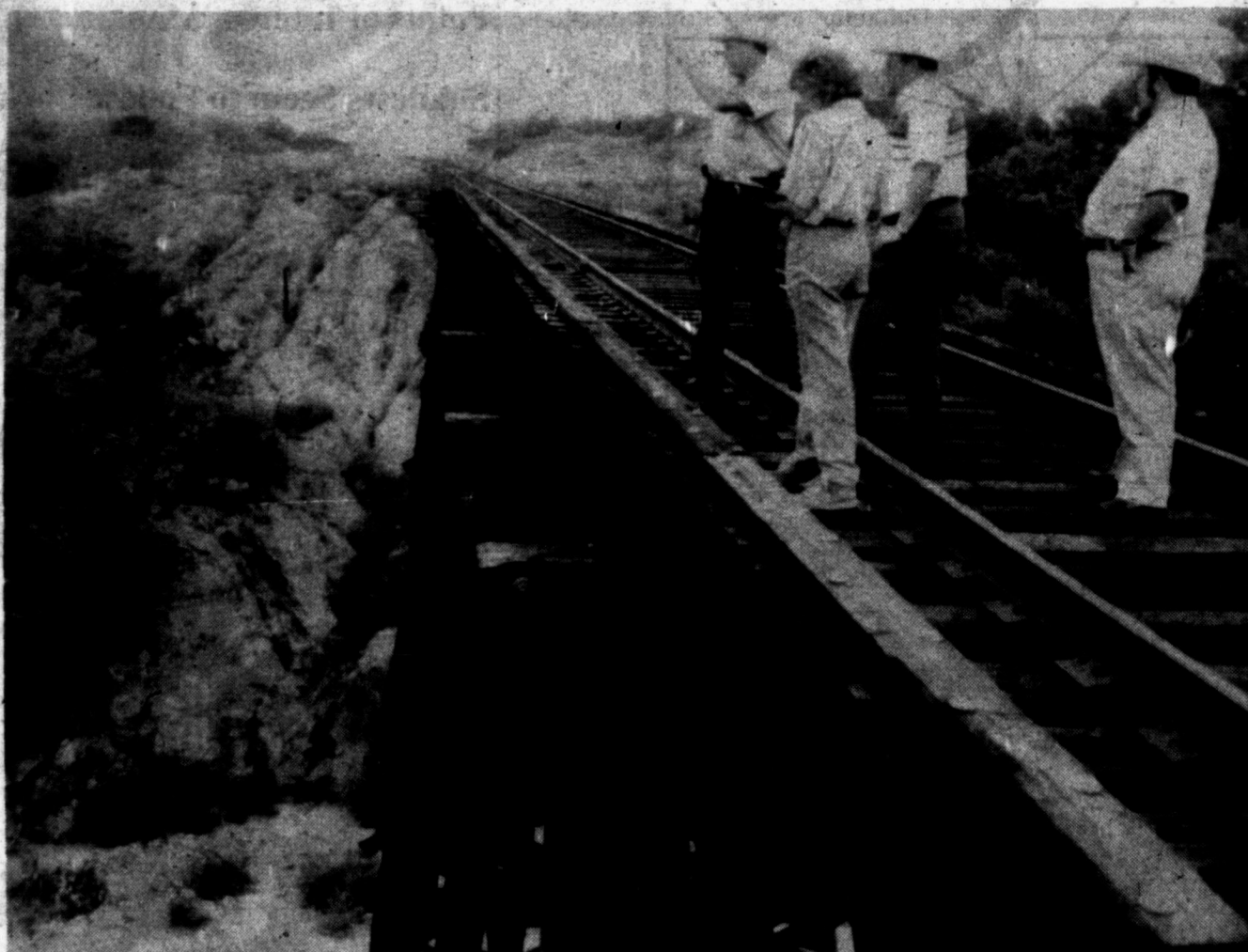
Community leaders and Texas Parks officials consider project plans from Caprock Canyons RR bridge.
