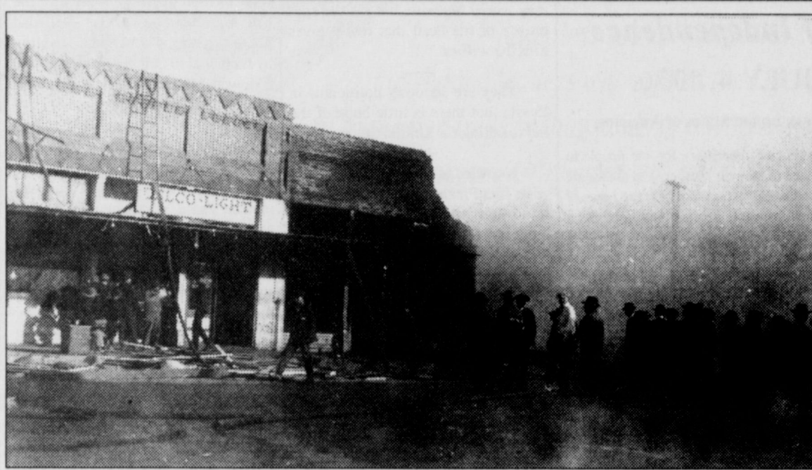
In late night hours of April 4, 1921, a storm ravaged Clarendon's business district which left several buildings in ruins. As far as we know, these photographs were not developed until the early 1930s and have never been published until now. Above is a picture depicting the damage done at the north end of Kearney Street by a bolt of lightning. The Delco-Light building on the left is still standing today next to the Mulkey Theater, but three buildings on its north side were destroyed, including the Couch restaurant and two grocery stores. Clarendon Office Supply and the abandoned Antro Hotel presently stand on these sites. Photos courtesy Helen Ann Parker.
