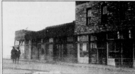
These buildings were located on the north end of Kearney Street and were on the east side of the street. They suffered heavy damage from the storm and were condemned by city officials.
