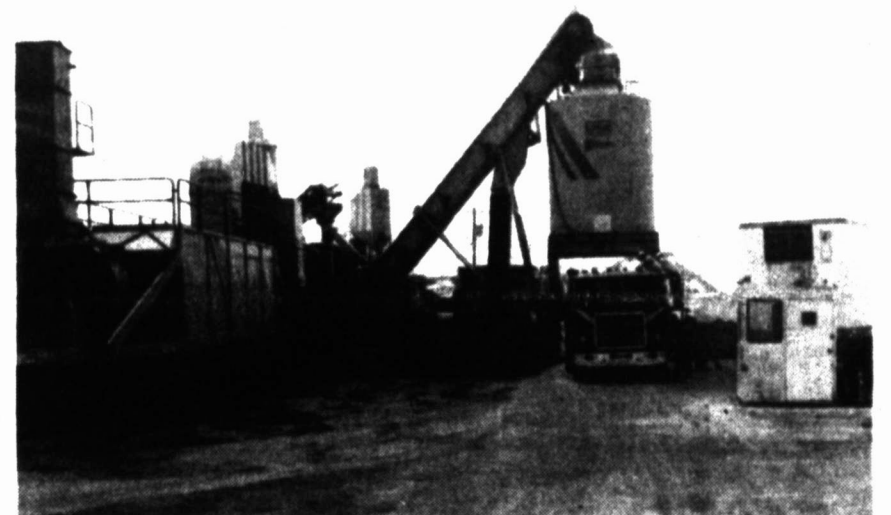
THIS BATCH PLANT is now in operation just east of Clarendon. It is producing paving materials for the renovation of the eastbound lane of Highway 287. Much of the passing lane between Clarendon and Hedley is blocked off for major repairs. Gilbert Construction is the contractor.
