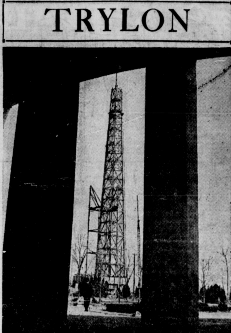
TRYLON NEW YORK—Using the massive columns of the Hall of Business Systems as a frame, a photographer caught this striking view on the site of the New York World's Fair 1939. The lowering steel skeleton is the Exposition's 700-foot Trylon, which will serve as Fair beacon and broadcasting tower. Directly in front may be seen the circular steel collar which will support the 200-foot Perisphere and the theme exhibit which will be housed within this great hall.
