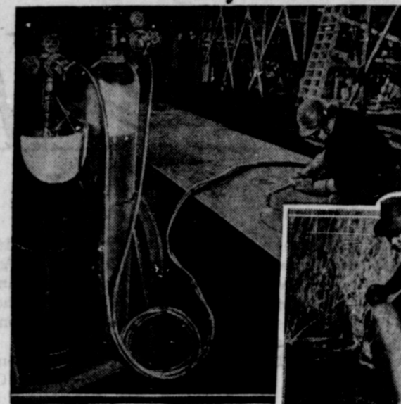
Above—Acetylene and oxygen cylinders at work in shipyard. They supply flame with which workers cut heavy metal as easily as housewife slices butter
