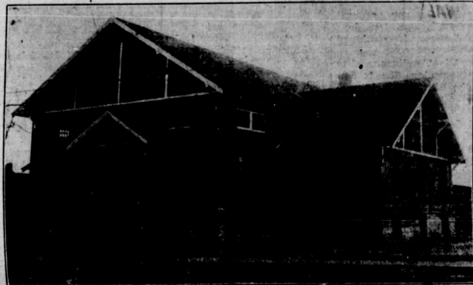
Clarendon's First Christian Church which was built about twenty-five years to serve the growing congregations. Rev. L. Guy Ament is now serving as pastor of the Church where services will be held Easter Morning. Rev. Ament is also holding revival services both morning and night.
