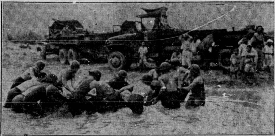
BATTLELINE STRUGGLE IS NOT ALL SHOOTING —U. S. Army Engineers use two-wheeled native cart to remove boulders from Korean river bed to open a ford for the advance of American motor vehicles.
