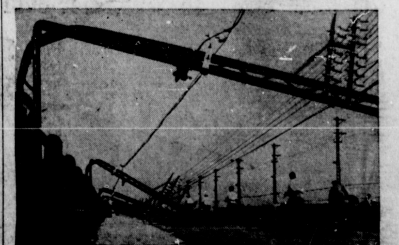
OSAKA, Japan—Pictured above are steel telephone poles twisted into fantastic shape on the Yodo bridge in the wake of the worst typhoon to hit the Kobe-Osaka area in 16 years. More than 100 died and 1,000 were injured in this hub of Japan's industry.
