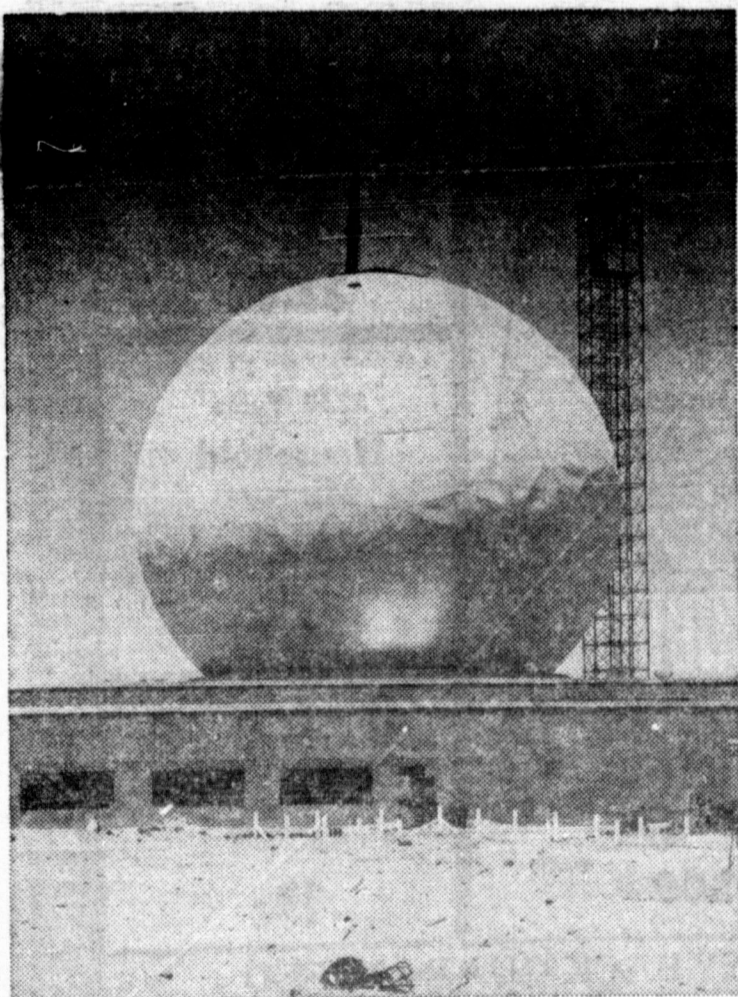
"SNOWBALL" IN NEW MEXICO—Towering above the desert at White Sands, New Mexico, is the experimental model of the modern U. S. Army's Nike Zeus acquisition radar being used in the current program of firings of early test models of the Army missile now in research and development stage. The Zeus is the only anti-missile missile in sight capable of defense against intercontinental ballistic missiles. Acquisition radar is used to locate and lock onto enemy missile and furnish firing data for the interception.
