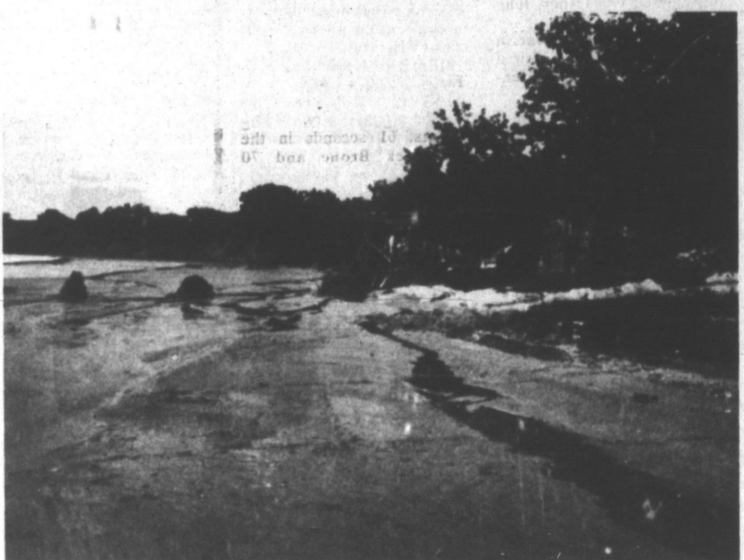
WHITEFISH BRIDGEOUT—This crossing to the Al Cooke Ranch was demolished during the recent flooding. Repair work throughout the area is underway by the county commissioners.
