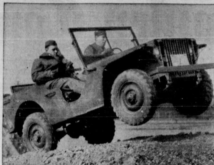
Speed shot at Camp Holabird, Maryland, during tests on new Light Reconnaissance and Command Cars for United States army. They carry machine gun and crew of three men at approximately 60 miles an hour. Can climb steeper hills than tanks. The Ford Motor Company, which built the ditch-jumper shown above, has an army order for 1500 of these units.
