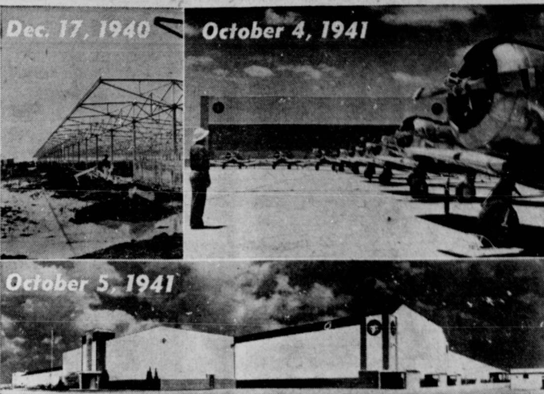
The above picture will give the reader some idea of plane production in the nation. This factory was completed in 120 days in Tarrant county. There is 25 acres under one roof. The building has no windows, a precaution against "black-outs", should the necessity arise.
