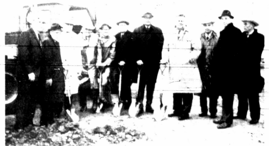
GROUNDBREAKING Ceremonies April 17, 1967 to begin construction of Greenbelt Reservoir. Present were Andy Rodgers, Clifford Johnson, Howard Boswell, Marvin Shubert, Bill Burger, Dr. S. H. Townsend, Wendell Harrison, Carroll Knorrpp, James R. Nichols, Wm. J. Lowe and J. M. "Red" Simpson. Photo Contributed
