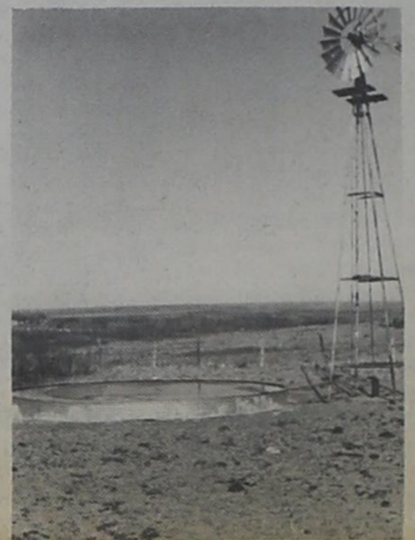
WELLS AND WATER STORAGE Facilities developed through the Great Plains Conservation Program are a source of abundant, high quality water for livestock on Donley County ranges. The water storage facility is designed to furnish adequate water for the maximum number of livestock watering at the facility for a period of seven days without additional water. This type of facility is used extensively in well managed grazing systems on lovegrass and with planned grazing systems on native range. This facility can also be used in conjunction with pipeline so that one well may better serve one or more pastures.
