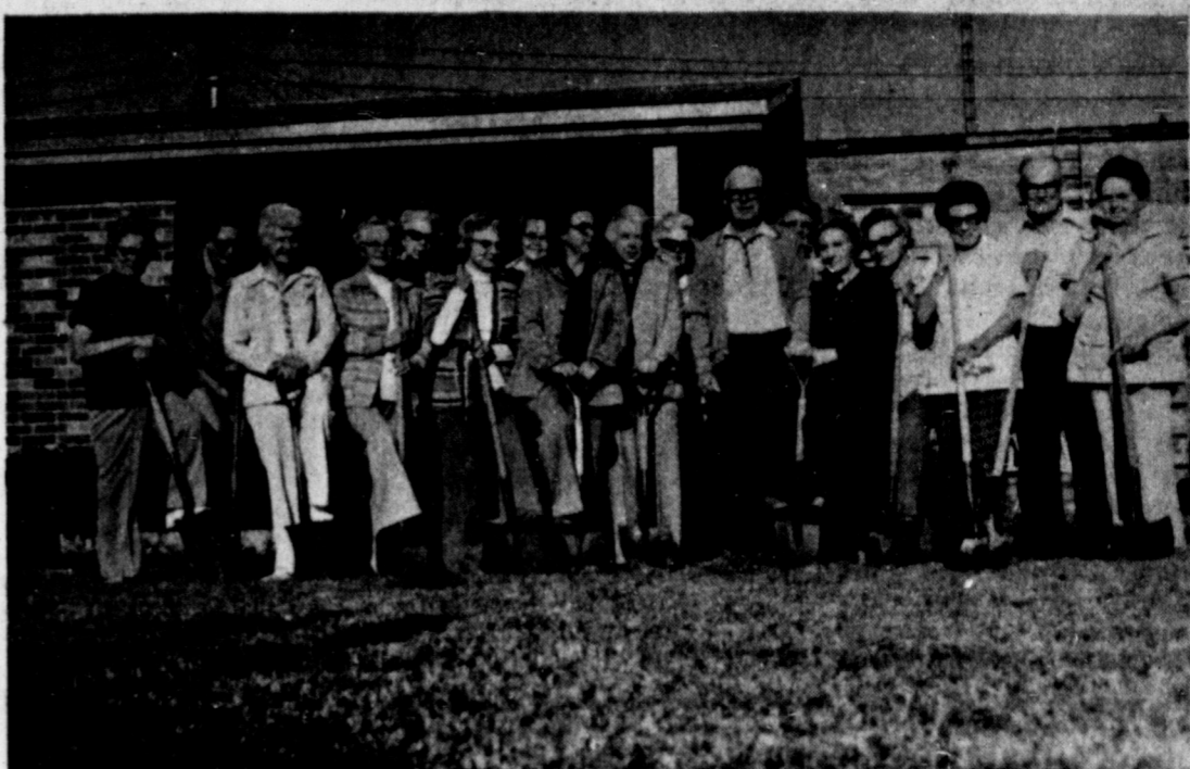
GROUNDBREAKING FOR THE addition to the Senior Citizens is also a team effort with everyone taking part.
