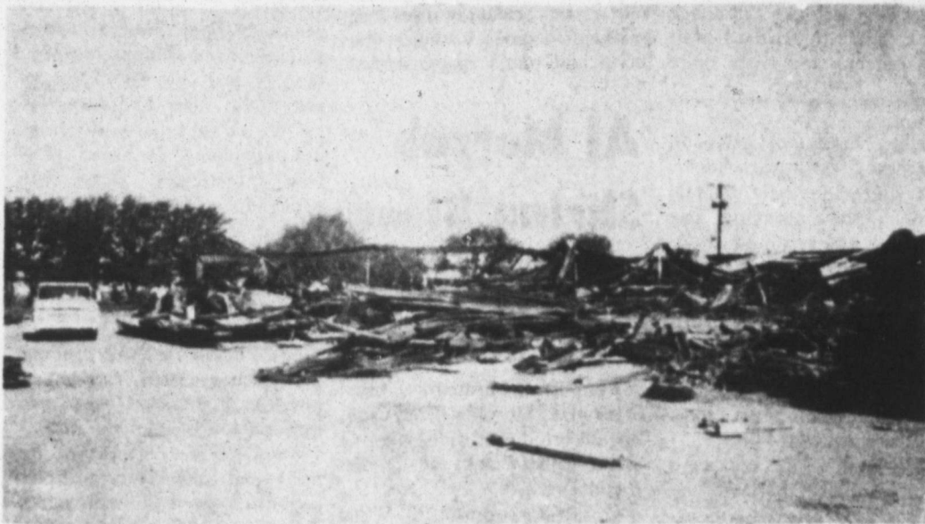
CLEAN UP JOB CONTINUES AT GIBSON'S
