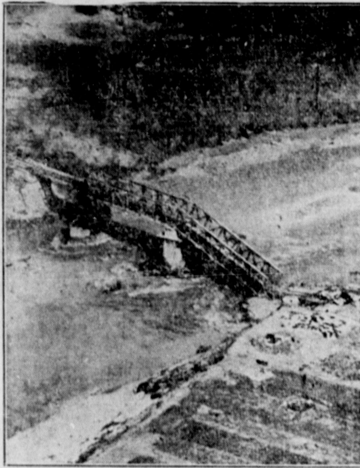
Released by U. S. War Department, Bureau of Public Relations. ON THE ENEMY'S SIDE OF THE MOUNTAINS —After units of the 15th Air Force received the go-ahead signal following a forecast of clear weather, U. S. planes soared over lofty peaks in northern Italy and smashed this German-held railroad bridge. Just one incident in the contribution to Nazi defeat.
