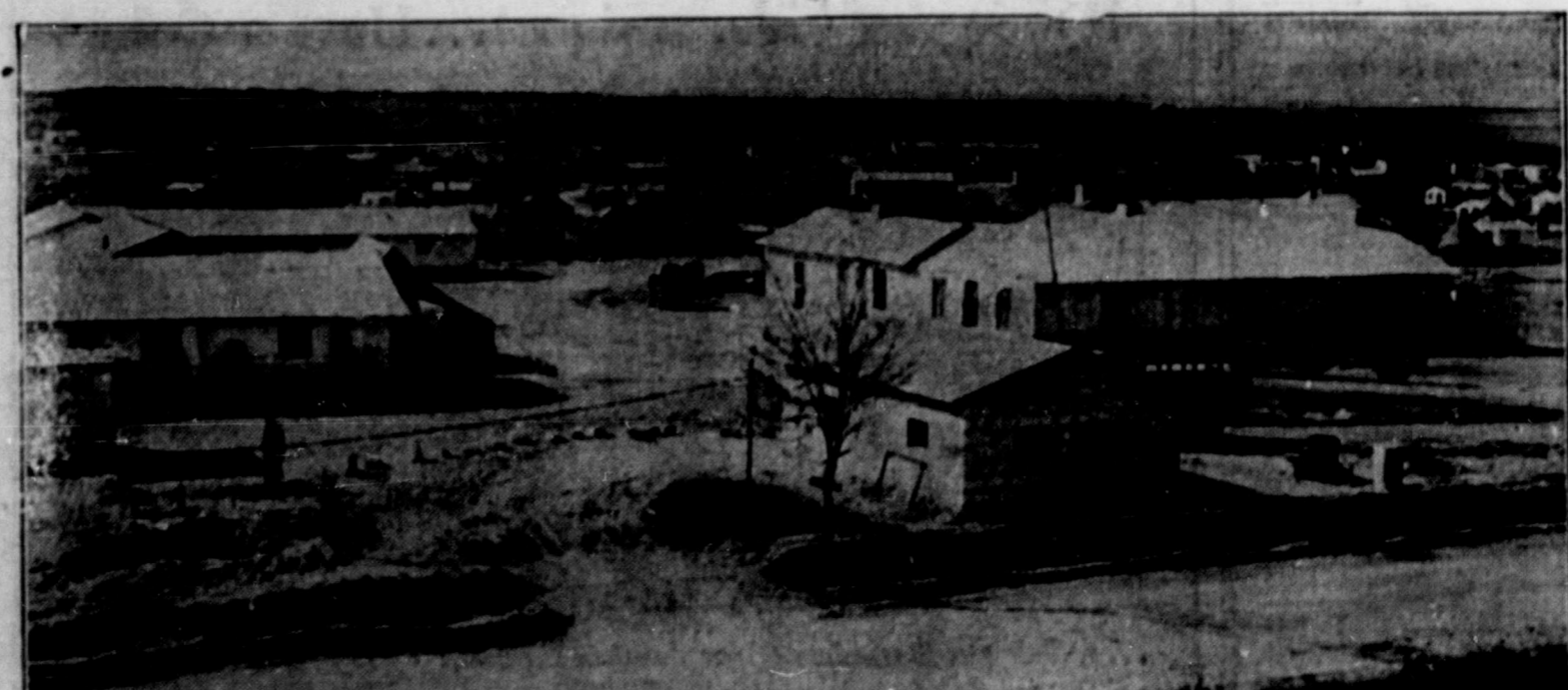
U. S. AIRMEN BUILD THEIR OWN VILLAGE—At a 15th Air Force heavy bomber base in Italy ingenious GIs resolved to "winterize" against the cold, rain and mud that hampered life in their tents. Building blocks of tufa stone were obtained at a few cents apiece, transportation was available, salvage material was abundant and there was no man power shortage insofar as architects, builders and decorators were concerned. They went to work with a will during off-duty hours and this town is the result. The investment in their villas ran from $30 for a one-room house to $200 for a six-room affair.
