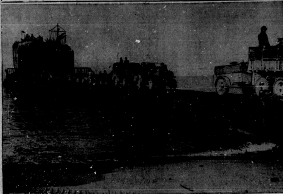
The Army engineers were on the job at Pesto, Italy, near Salerno, when Lieut. Gen. Mark W. Clark's invaders landed on Hitler's Fortress Europa. Here you see a pontoon dock, where one of our big landing craft is unloading, laid right to the beach. Some idea of the size of these new landing boats built for invasions such as that of Italy can be made by comparing it with the trucks that have been swarming out of its giant maw. Your War Bond purchases helped to build such landing craft and those trucks.
